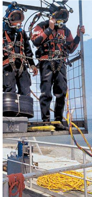
Installation of AMEX®-10 MONO Seal with divers in a flooded pipe system
