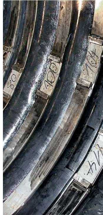
Detail showing a AMEX®-10 VARIO installation under strong water pressure from outside
