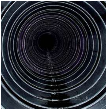
Sealing of a pressure pipe diameter 1800 with AMEX®-10 VARIO System
