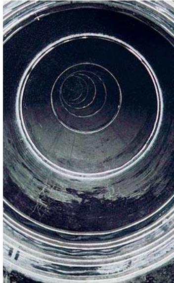
Partial sealing with AMEX®-10 VARIO System
