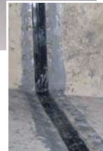
Sealing of a construction joint in a container for potable water, corner shaped, with AMEX ® -10 MONO Seal
