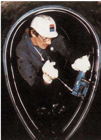
Installation of AMEX®-10 MONO Seal in an egg shaped sewer
