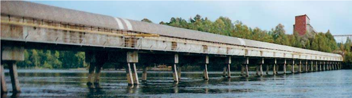
Sealing of a pipe running across a bridge in Scandinavia with AMEX ® -10 Internal Sealing System, temperature range: -30 °C to + 25 °C.
