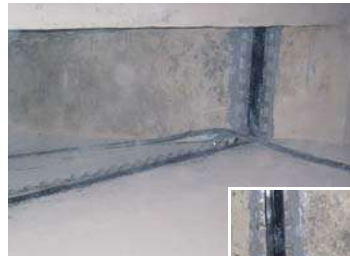
Sealing of a construction joint in a container for potable water, corner shaped, with AMEX ® -10 MONO Seal
